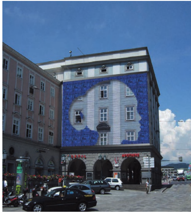
Figure 4. The Solar Display in the layering function. The original facade is still visible while only parts of the facade are being used for display functions.
